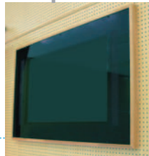
▲ For some sports, a cover is mounted on the front screen, or the entire display is embedded in the wall, to protect the athletes from possible accidents.
